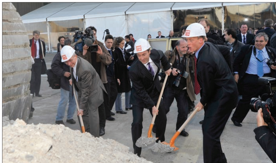
The start-up of construction for the A350 XWB final assembly line in Toulouse was marked by a symbolic groundbreaking with Airbus officials on January 14.
