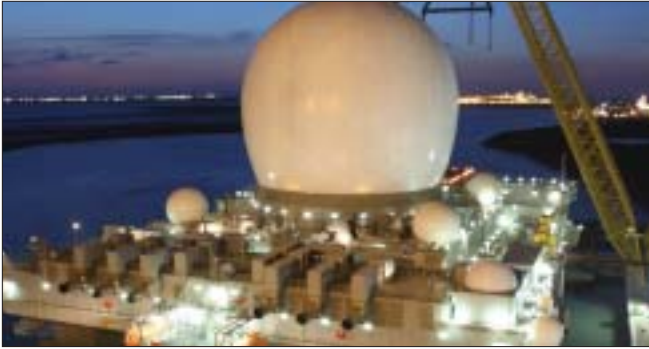
The SBX radar, seen here on a mobile oil rig, is 27 stories high.
