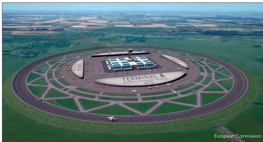
Circular runways, as in this artist’s rendering, would take up less land and offer shorter taxi times than conventional runways. But pilots might take awhile to feel comfortable landing and taking off while turning on a bend.
