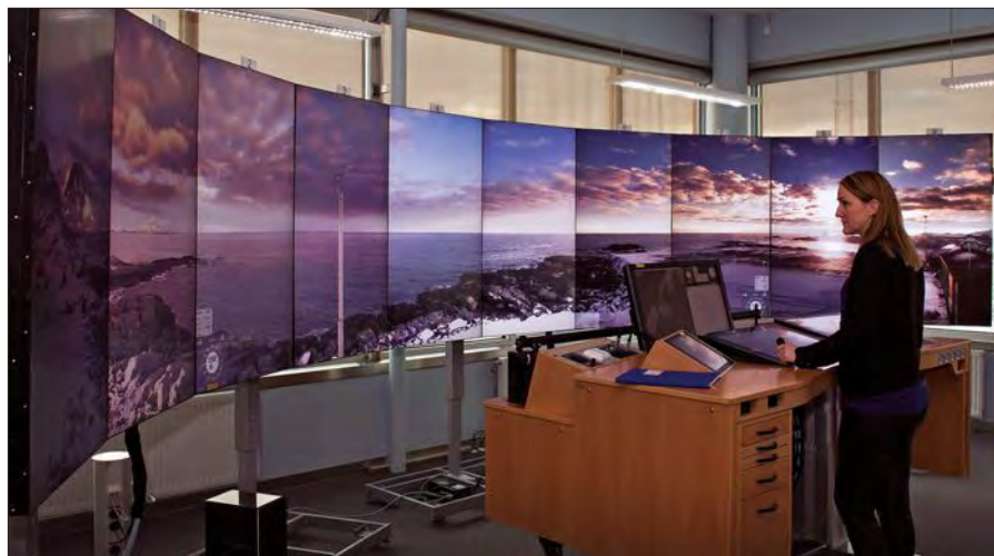
A panoramic screen shows traffic at an airfield far away from Norway's Bodø Airport, where remote towers have been tested.
