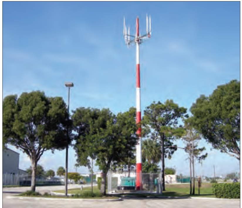
This ADS-B ground station is located in southern Florida. (Photo courtesy ITT.)
