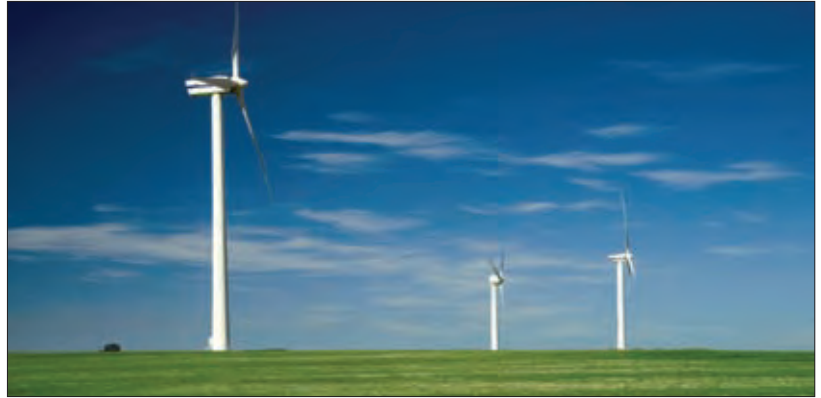
Eskom is developing wind farms in the Western Cape in South Africa.
