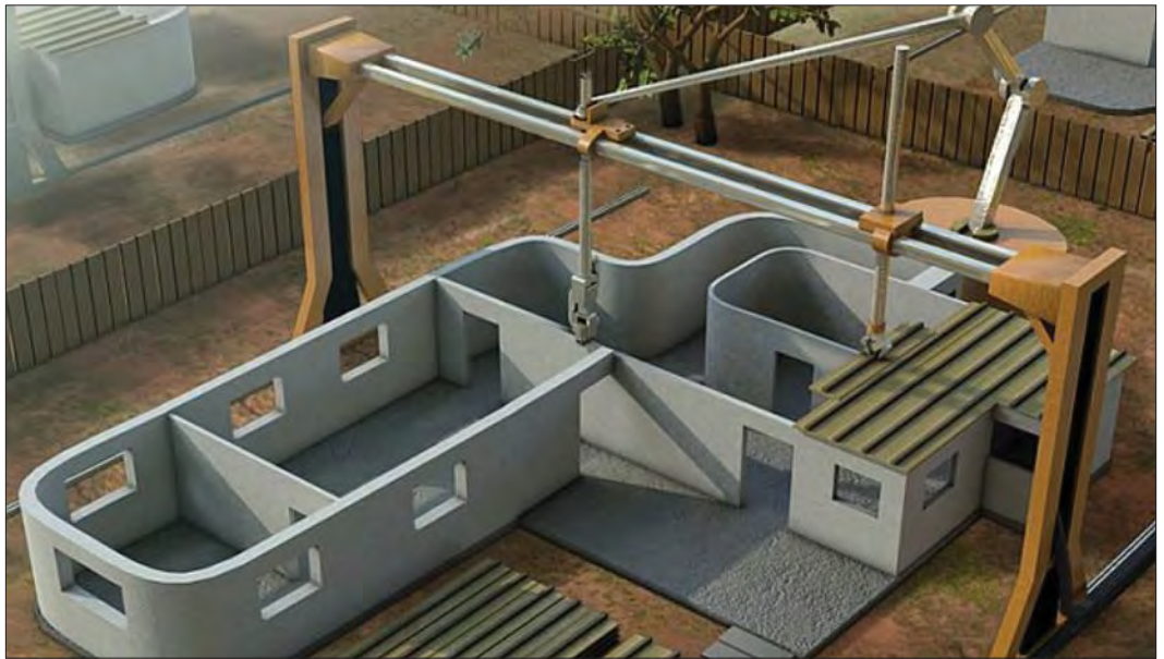
Print your house: The Contour Crafting machine developed at the University of Southern California releases quick-setting concrete to build structures layer by layer. The method could someday be used to build huge structures on the moon.
