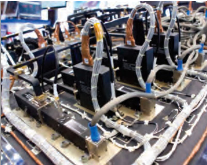
A satellite communications payload shows traveling wave tubes and electronic power conditioners. Credit: Mark Williamson.
