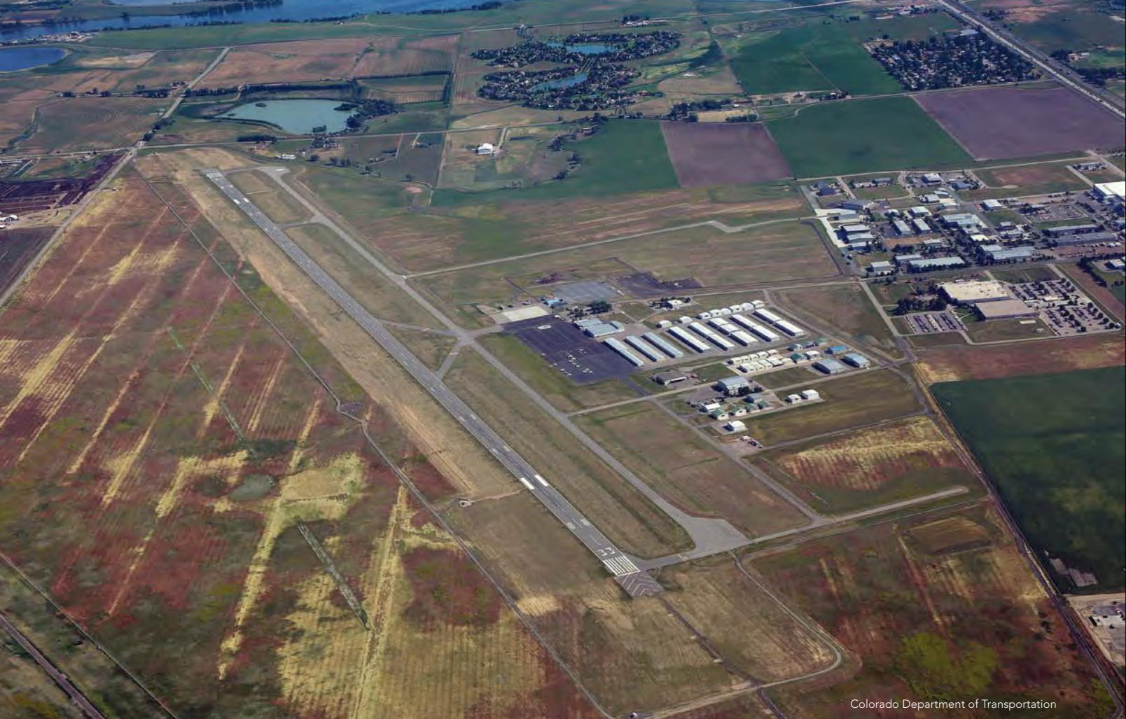
Offsite air traffic control: Loveland-Fort Collins Airport in Colorado does not have a physical control tower, so it plans to feed video and data from sensors in mountain passes to controllers at another location.
