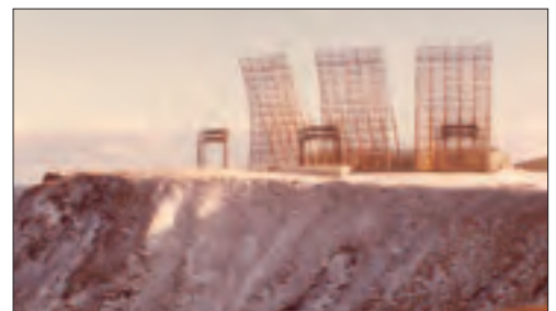
The FPS-17 radar system rests on the island of Shemya, Alaska. This version of the radar was used to detect the final phase of missile tests launched from Tyuratam. With several added antenna elements, this version of the FPS-17 covered four times the area covered by the system installed at Diyarbakir, Turkey. Courtesy James Moss.
