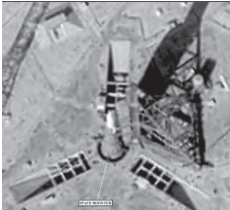
A GAMBIT 3 photo shows the SL-X on its launch pad at Area J on September 19, 1968. The blast pit deflectors and the service gantry tower are easily seen. The pointed-tip shadow of the rocket itself is directly behind the launch vehicle. This close-up image was released by the NRO in January 2012. At the time of the release, decision-making on how clear to make the specific GAMBIT 3 images released to the public was still in flux. In this individual case, a decision was made to electronically ‘de-focus’ the image so that the true capabilities of the imaging system would remain hidden. Courtesy NRO.
