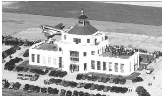
The 1940 Air Terminal on Opening Day, at what is now William P. Hobby Airport in Houston.
