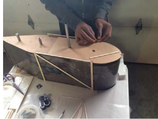
Figure 6-2: Fuselage Construction with Mold
